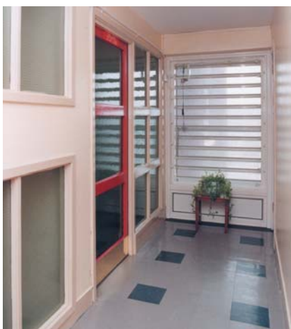
The EN Stairwell ventilator can be installed either vertically or horizontally, and is equally as effective as a corridor ventilator.
