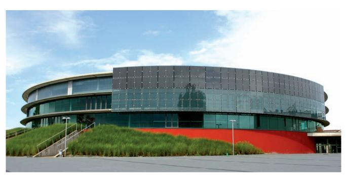
EWE Arena, Oldenburg, Gemany - Colt designed and suplied a movable solar wall complete with photovoltaic cells to provide both solar shading and the generation of electricity
