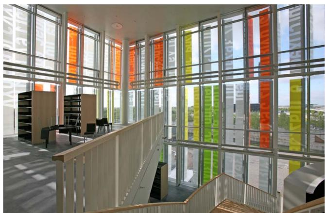
Ørestandens Gymnasium, Copenhagen, Denmark. - Colt designed and installed 700 laminated and printed bespoke Shadoglass glass louvres over an area of 1700m² of façade for shading and ventilation. The different colours, films and frits provide a youthful and playful appearance.
