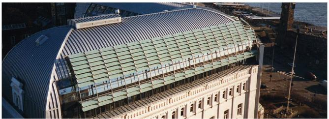
Hotel Hafen, Hamburg - Fritted glass louvre system, enabling daylight to enter the building through the roof whilst reducing solar heat gain
